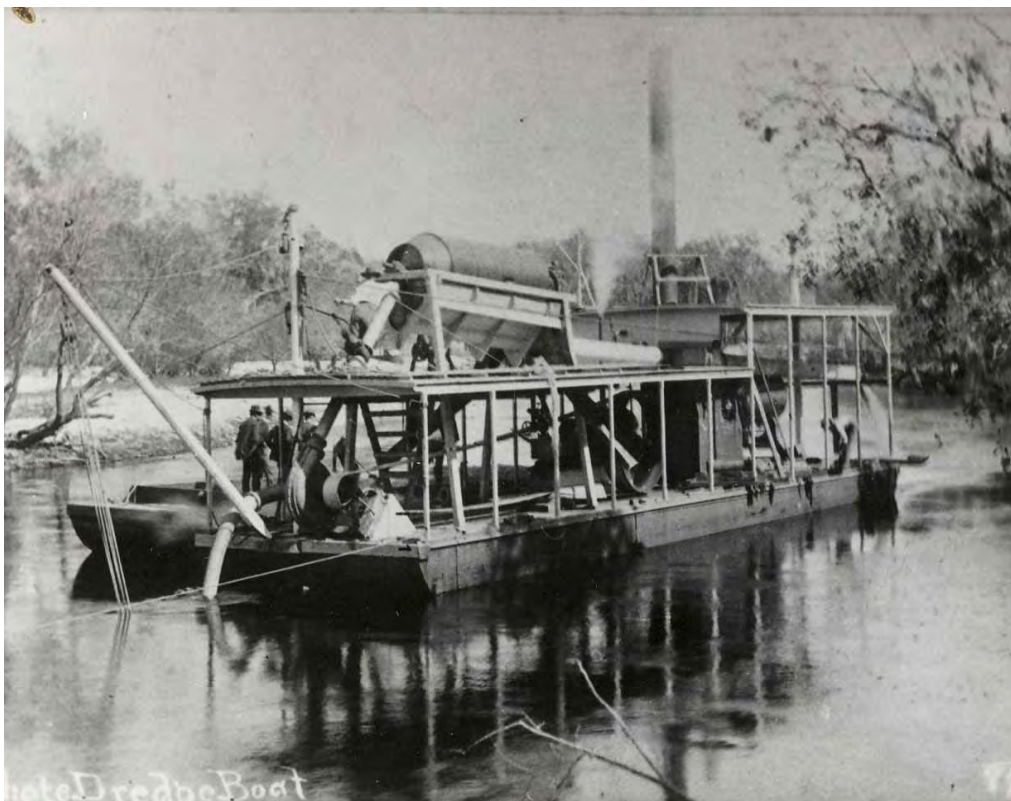
River Pebble Mining on the Peace River Using a Suction Dredge, ca. 1895
